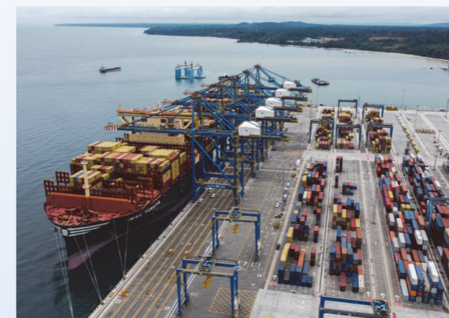
Wharf of Kribi Deepwater Port Phase II in Cameroon
