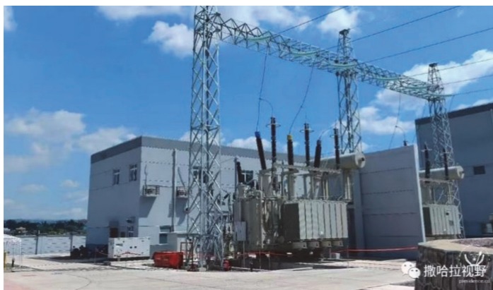
The 220kV Kinsuka Substation Project in DRC
