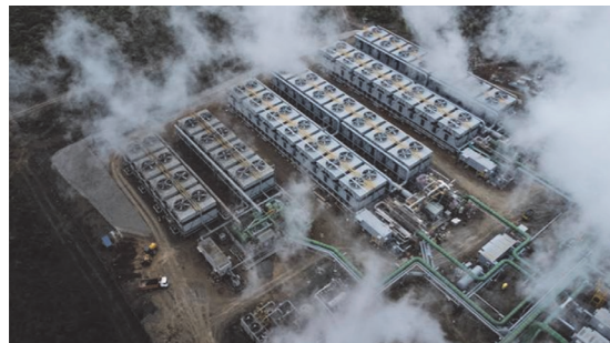
Construction site of Suswa Geothermal Power Station in Nakuru, Kenya
