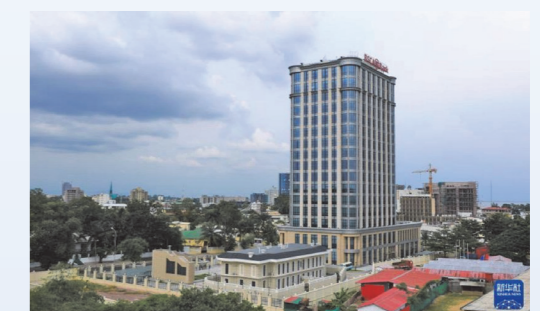
The office building of Bank of Sino-Congolese Bank for Africa (BSCA), located in Brazzaville, the capital of the Republic of Congo
