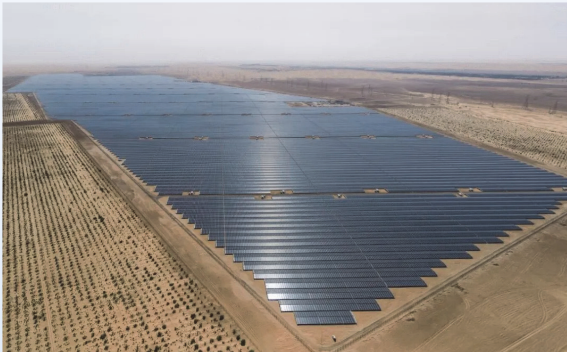
Solar Power Plant in M'Ghair Province, Algeria
