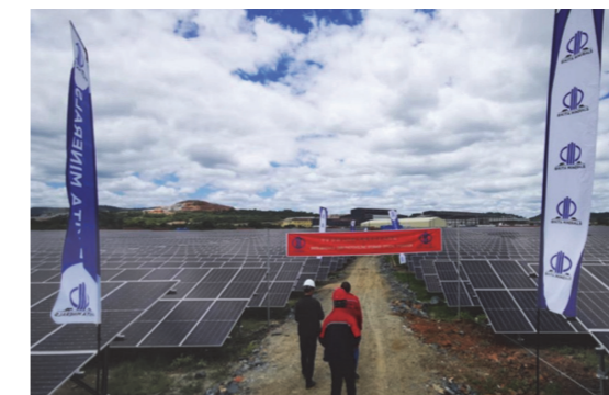
Photovoltaic power plant at Sinomine Bikita Mine
