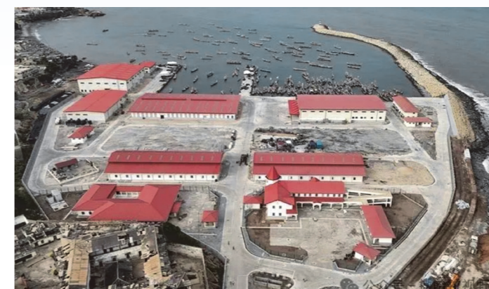
China-aided Fishing Port Complex Project in Ghana
